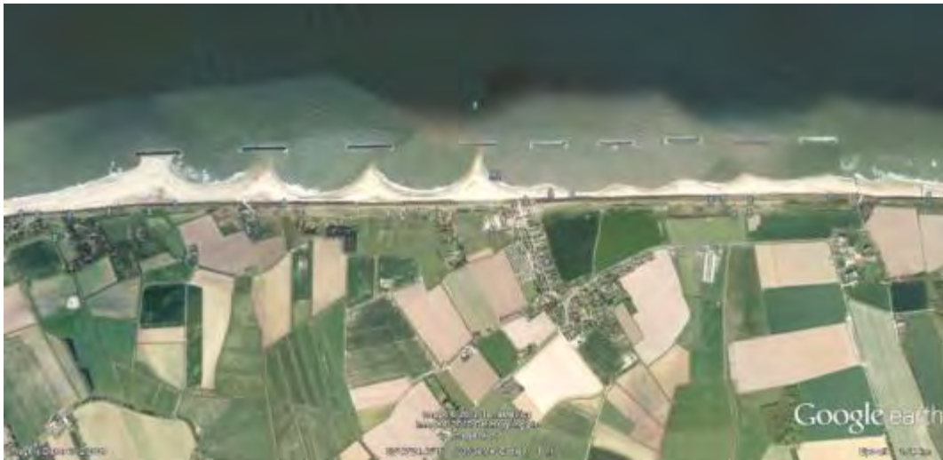
Breakwater scheme at Sea Palling, Norfolk, UK
