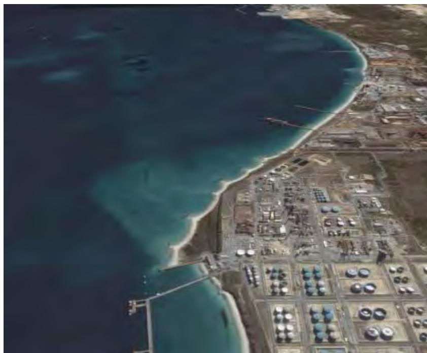
Use of headlands to stop sand incursion into a cooling-water intake since 1981
