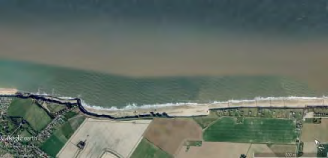
Existing eroding coastline at Happisburgh, Norfolk, UK
