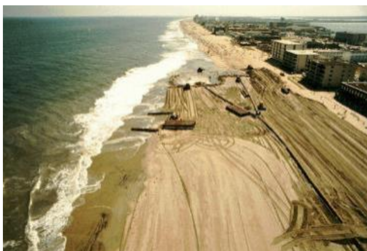
Beach replenishment at New Jersey, USA
